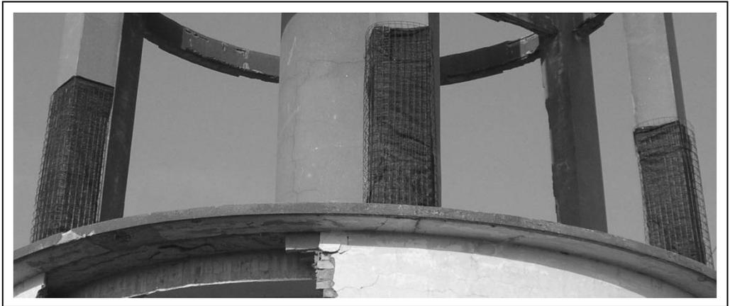
Figure 7. Wrapping of concrete pillars with steel mesh and textile.
