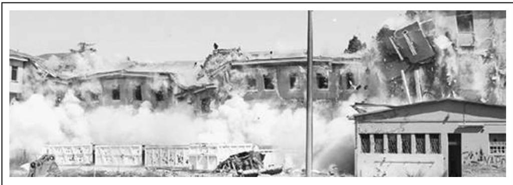
Figure 5. Blasting demolition of school building in thickly populated area.
