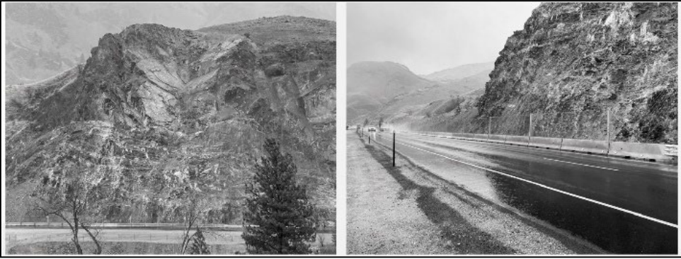
Figure 17. Completed mitigation of the rockslope, rockfall fence and US-95 highway, December 2020.
