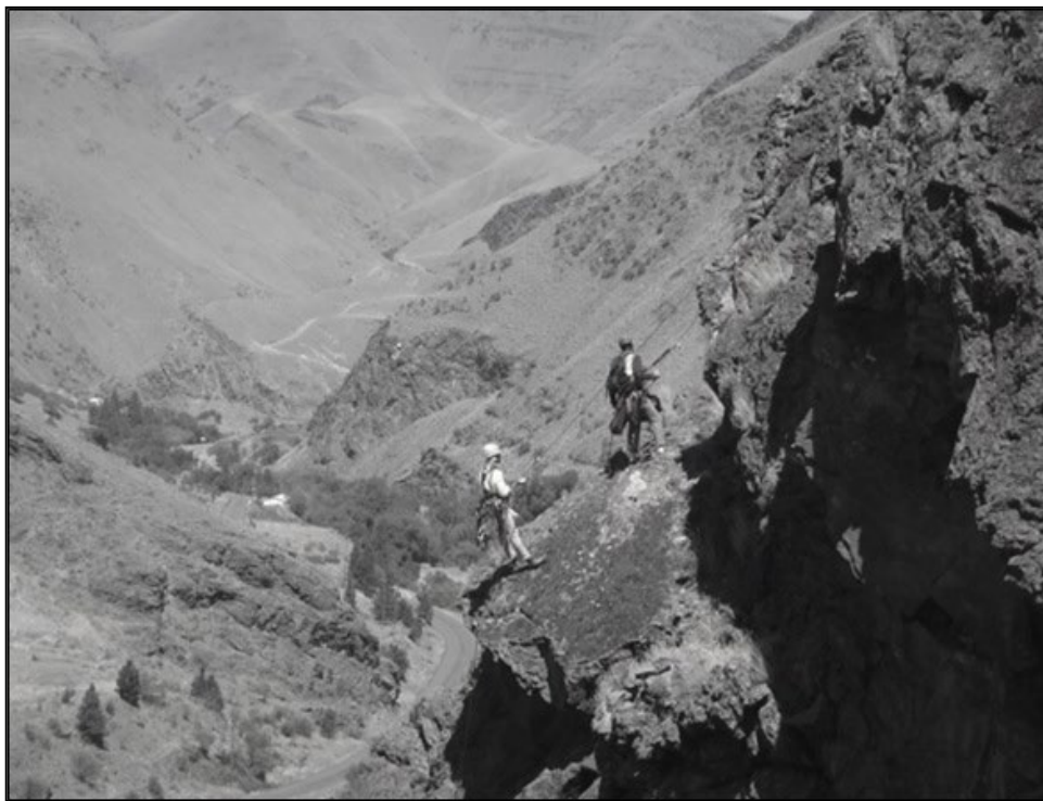
Figure 16. Ethan Guzek and Luke Ferguson with MJA assessing the stability of the rockslope using rope access safety techniques after the primary blast on 28 August 2020.
