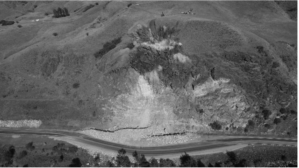
Figure 14. The Shot at 1730 hours on 28 August 2020. Note the catchment berms at the toe of the slope.
