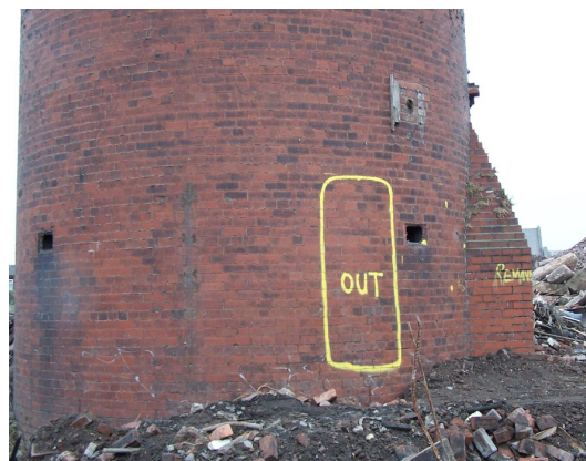
Preliminary Setting out of Openings in Masonry Chimney
