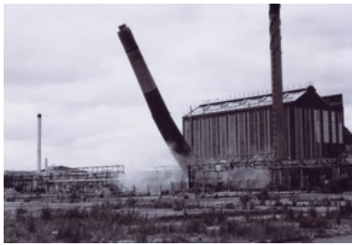
Masonry Chimney Widnes
