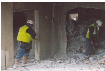
Wall Drilling to RC Walls
