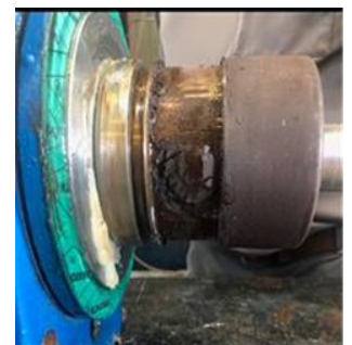
Emulsion/grease mix inside Joint
